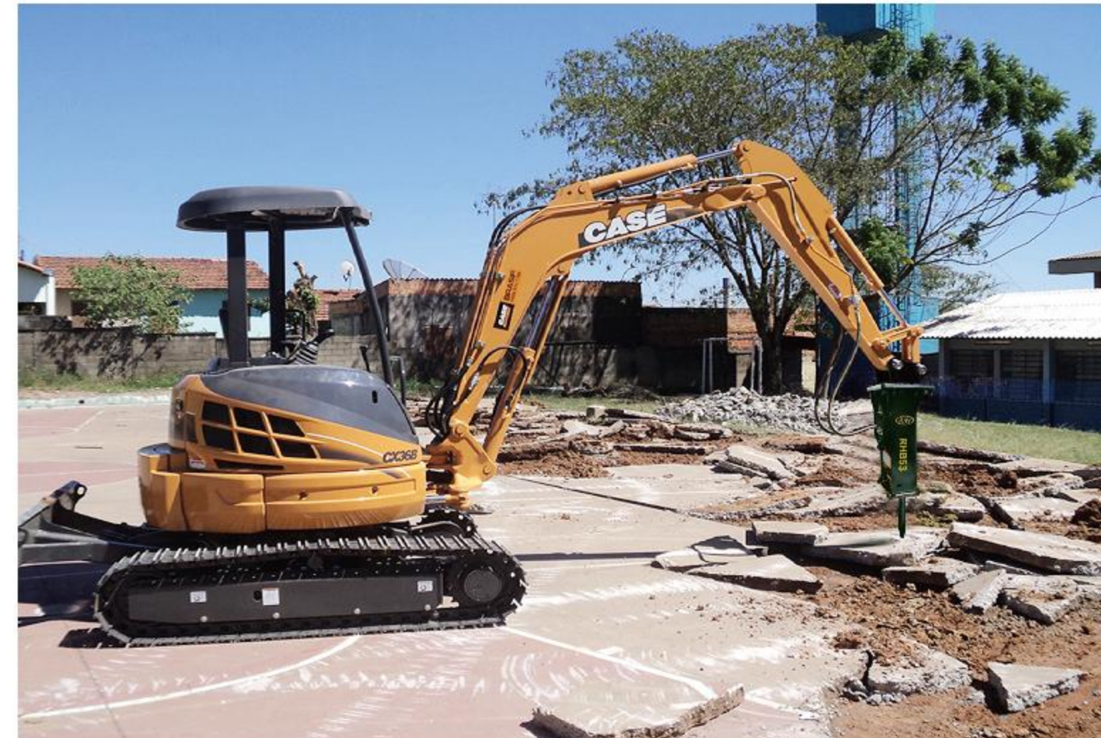
Skid steer loader : CASE CX36 Hydraulic breaker: RHB53 Box silence type Country: New Zealand
